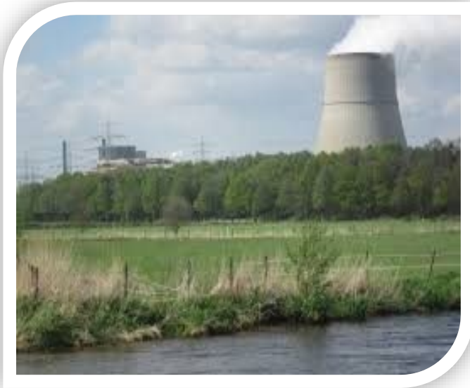
When it was decided that the Lingen prototype BWR should be decommissioned, Canadian expertise was deployed to plan the segmentation of the reactor vessel.
