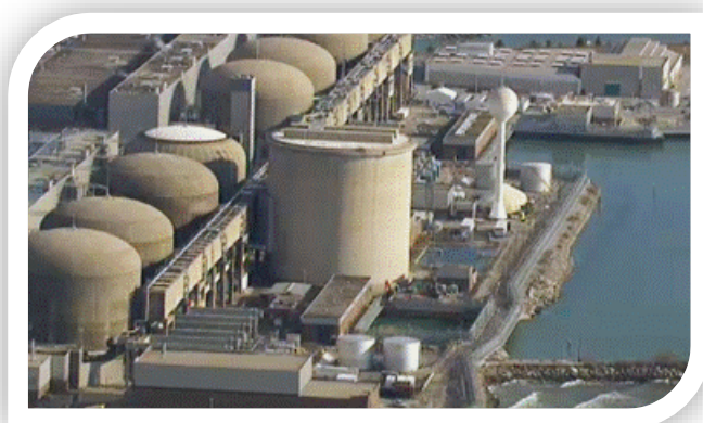
The Pickering Nuclear Generating Station will be the largest such decommissioning project in the world
